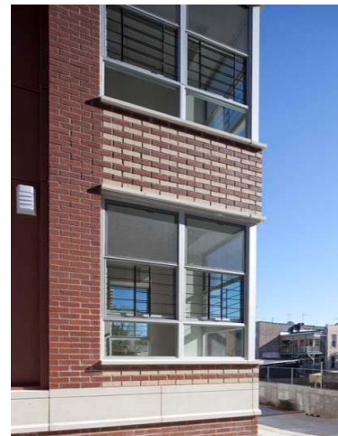
NORTHEAST CORNER WINDOW COMPLETED CONSTRUCTION
