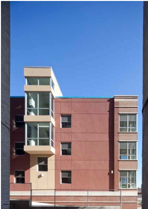
PARTIAL NORTH FACADE COMPLETED CONSTRUCTION
