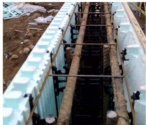
ICF PLAN VIEW WITH RE-BARS DURING CONSTRUCTION
