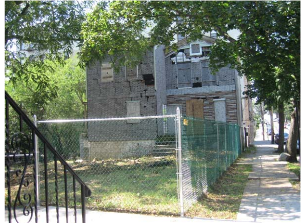
SIDE VIEW OF BUILDING LOT PRIOR TO CONSTRUCTION
