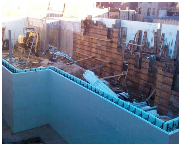
ICF FOUNDATION AND STANDARD FORMS DURING CONSTRUCTION
