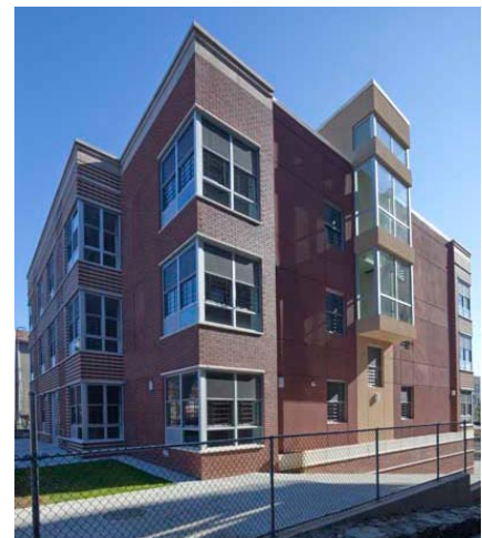
NORTHEAST FACADES COMPLETED CONSTRUCTION
