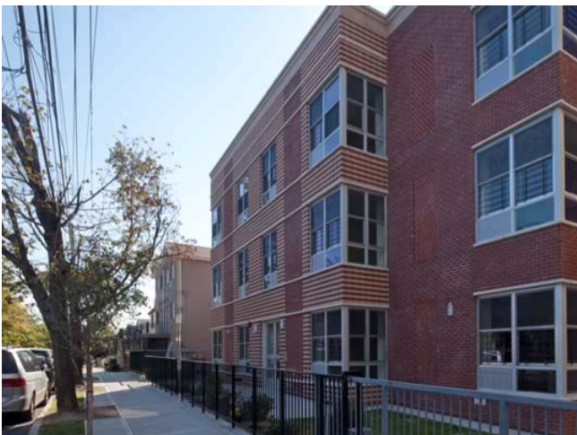
VIEW OF FRONT FACADE CONSTRUCTION COMPLETED
