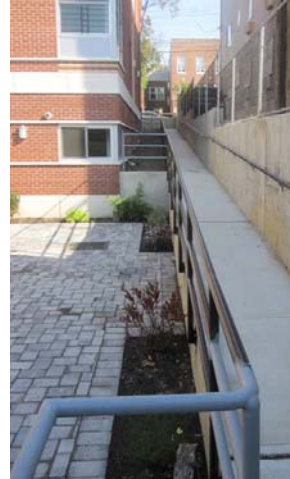
VIEW OF SIDE YARD WITH ACCESS RAMP DURING CONSTRUCTION
