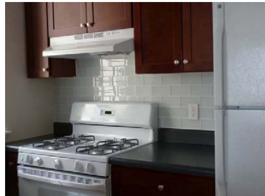
KITCHEN WITH ENERGY STAR APPLIANCES COMPLETED CONSTRUCTION
