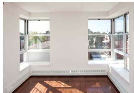
LIVING ROOM CORNER WINDOWS COMPLETED CONSTRUCTION
