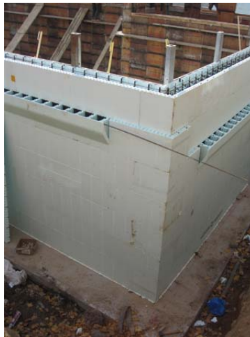
ICF FORM WORK DURING CONSTRUCTION
