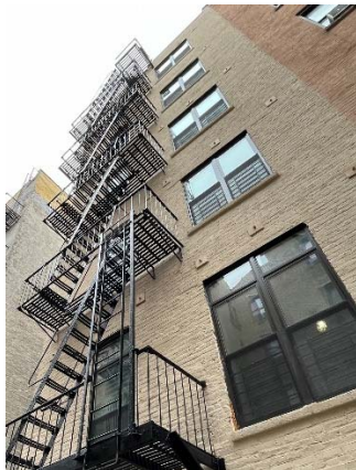
THROUGH ROD MASONRY TIES INSTALLED AT EXTERIOR WALL
