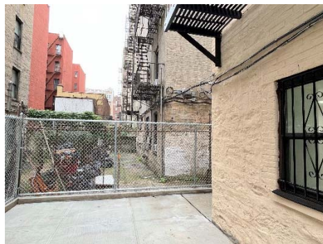
New concrete slab on grade in inner yard
