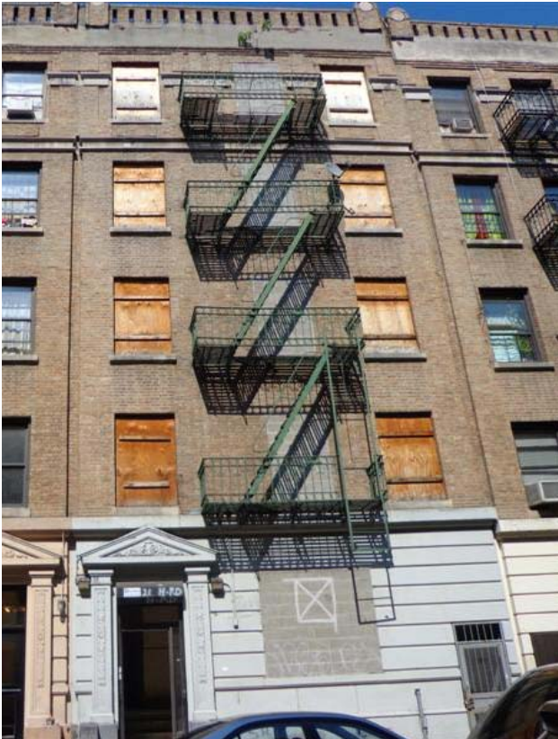
EXISTING BUILDING PRIOR TO RENOVATION
