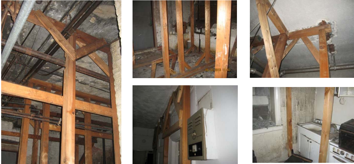
Images of temporary timber supporting each floor
