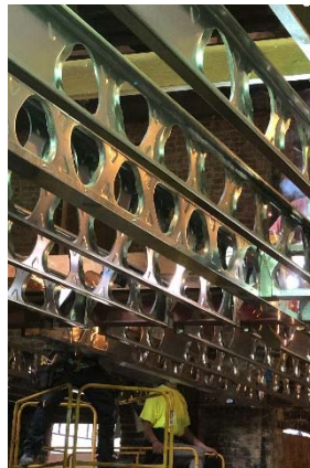
INSTALLATION OF JOISTRITE FLOOR JOISTS
