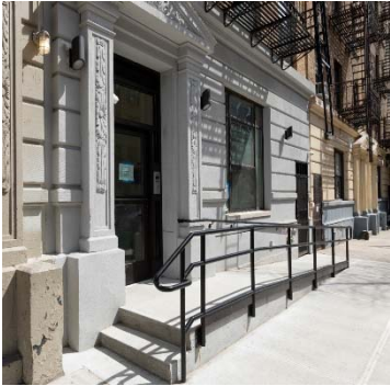
Handicap entrance ramp
