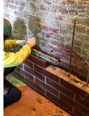
INSTALLATION OF STRUCTURAL ATLAS WALL
