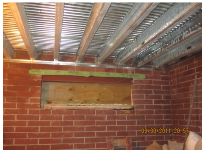
Steel frame joist system and atlas bearing wall Under Construction
