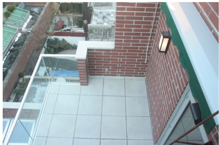
Atlas face brick bearing wall Completed Construction
