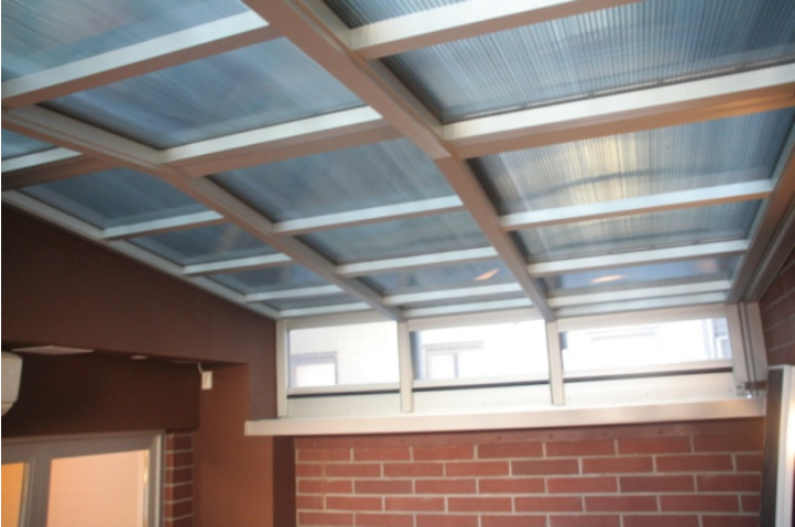
Retractable skylight above terrace Completed Construction
