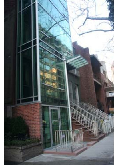
Townhouse entrances Completed construction
