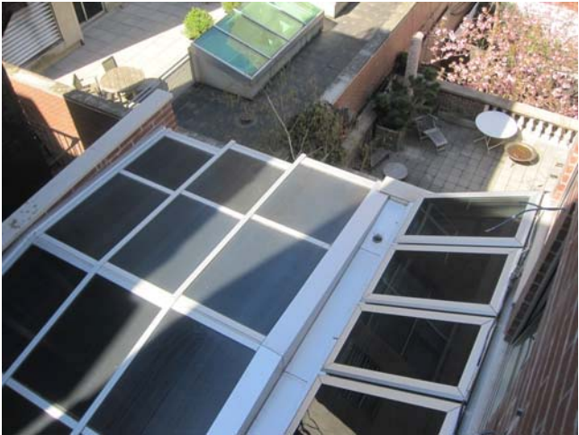
View of retractable skylight above terrace Completed Construction
