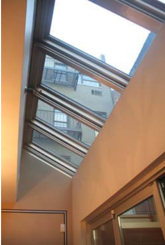
Operable skylight above bedroom Completed Construction
