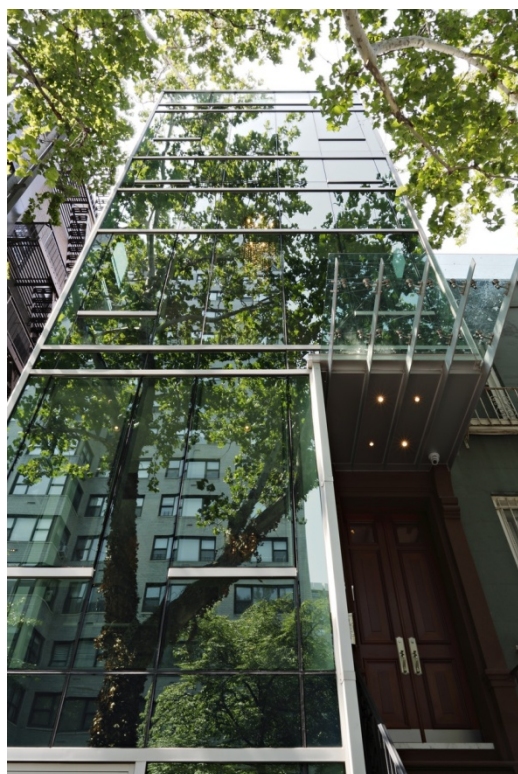
Completed Construction North Facade
