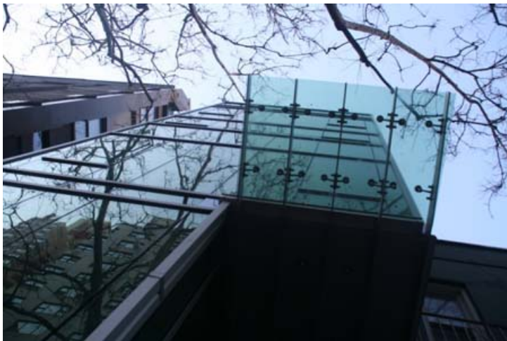
Curtain wall facade Completed construction
