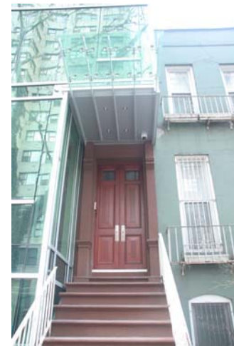
Entrance stoop stairway Completed construction
