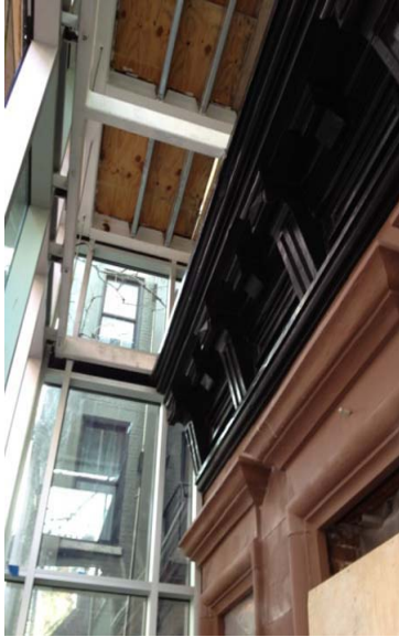
Existing cornice and enclosed porch under construction
