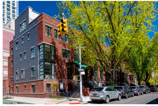
PARTIAL VIEW OF THE CORNER TOWNHOUSE LOOKING NORTH EAST
