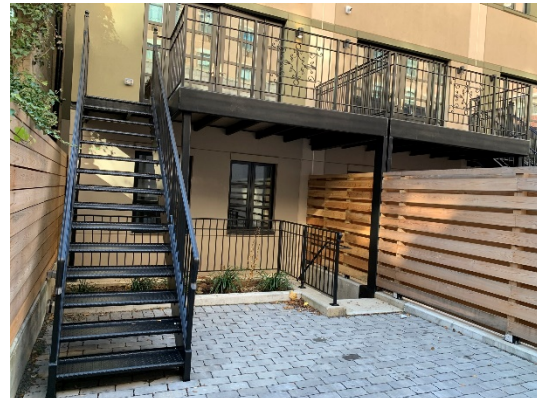
OUTDOOR DECK OFF KICTHEN LEADING TO BACK YARD
