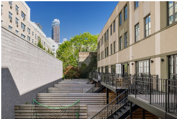
NORTH FAÇADE WITH EIFS SYSTEM
