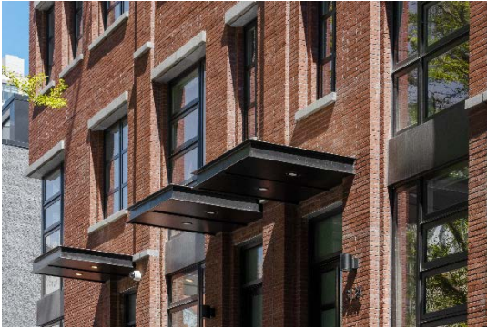
PARTIAL VIEW OF TOWNHOUSE ENTRANCES LOOKING WEST
