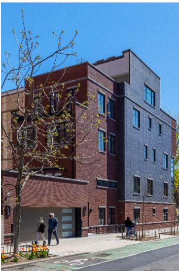
VIEW OF PRIVATE GARAGE OF 311 STATE STREET TOWNHOUSE FROM HOYT STREET
